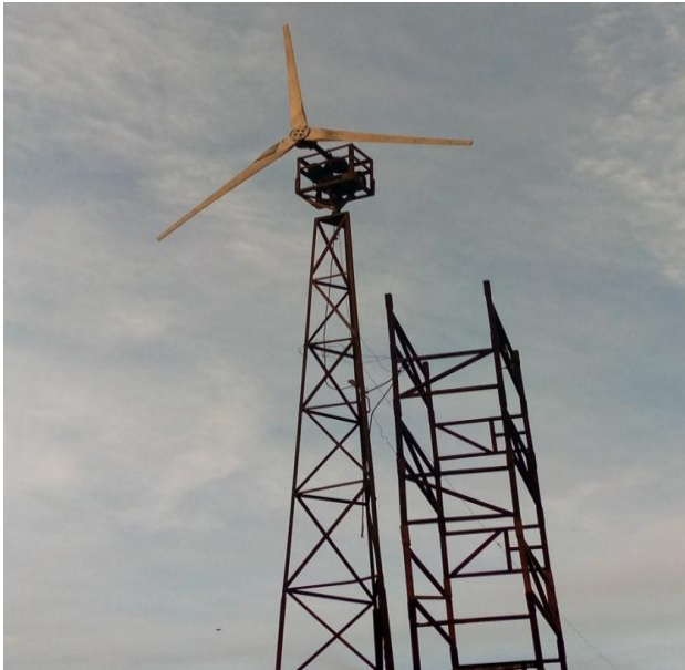
Source: photo NGAGOUM NITCHEU Vannelle, 2021 Photo7: Wind turbine installation
